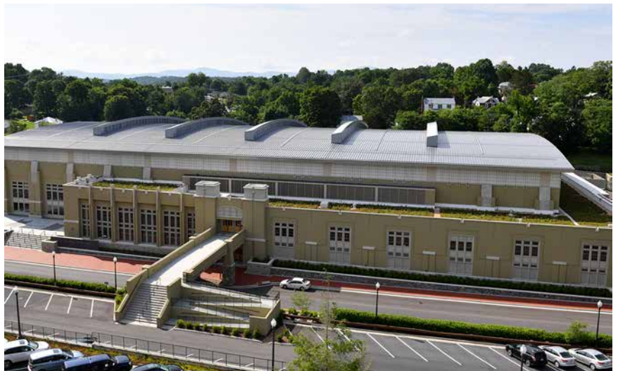
The green roof, which spans the lower two sides of the CPTF, slows storm water runoff and helps insulate the facility.—VMI File Photo by Kelly Nye.
