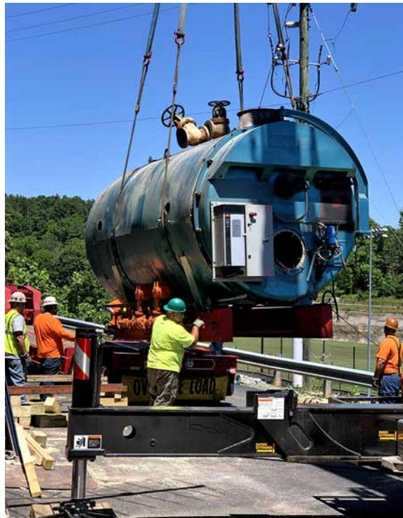
Crews remove one of the boilers from the heat plant on Burma Road earlier this summer.—Photo courtesy of Scottie Swisher.
