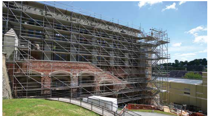
Underlying brick is exposed on Jackson Memorial Hall as new stucco is applied.—VMI Photo by Maj. John Robertson IV.
