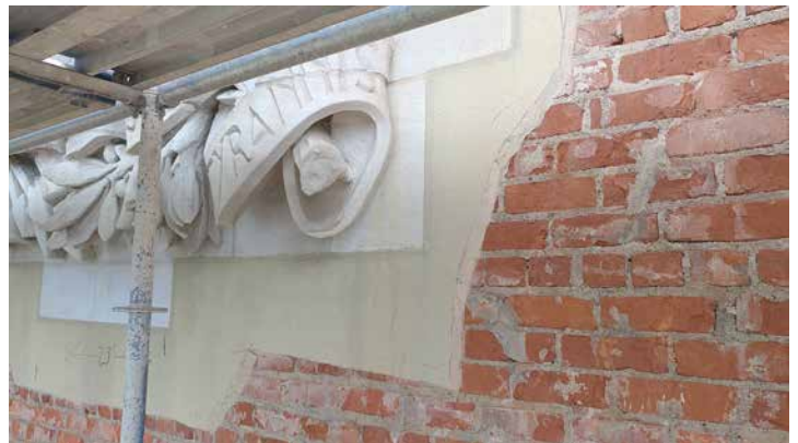
Damaged stucco was stripped down to the underlying brick wall during the repairs to Jackson Memorial Hall.—Photo courtesy of Maj. Michelle Caruthers.
