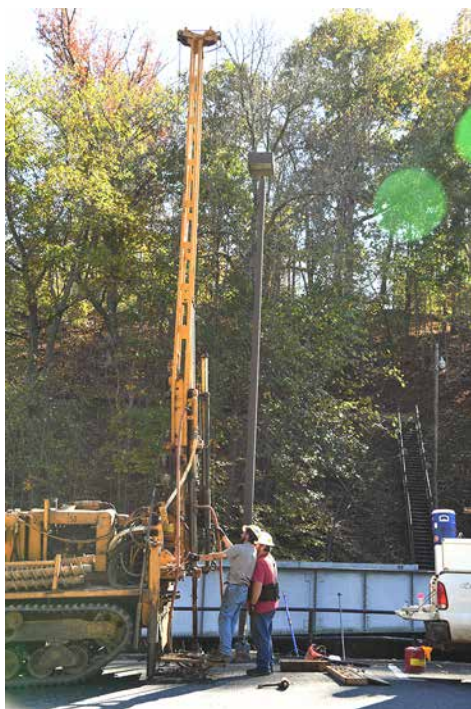
Drilling began on Oct. 24 to test the feasibility of widening Anderson Drive as part of the Post Infrastructure Improvement Project.—VMI Photo by H. Lockwood McLaughlin.
