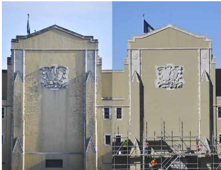
Cracks in the stucco on the back of Jackson Memorial Hall (left) are repaired after a four month restoration project (right).—VMI composite by Kelly Nye.
