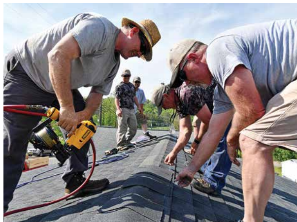
Physical plant members reshingle the roof of Buddy Lawhorn in Buena Vista on April 28. – VMI Photo by H. Lockwood McLaughlin.
