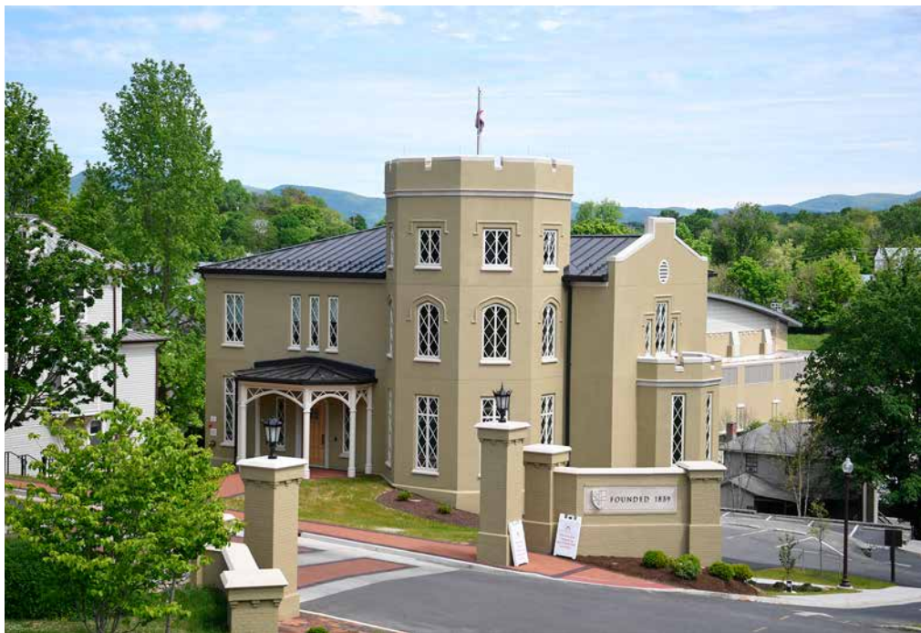
VMI Police are now located in a new headquarters on Letcher Avenue.—VMI Photo by Kelly Nye.
